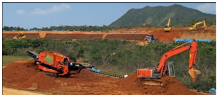
Large-scale Excavation and Sifting during Range Maintenance
