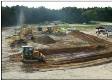
Backfilling the Infiltration Basin and the Storm Pipe System
