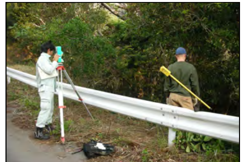
Surveyors Plot the Transects for UXO Avoidance During Construction
