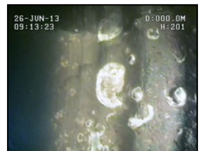
(above) Visual ROV inspection of sonar target; (below) calcified growth/shell on culvert wall
