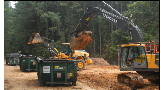
(top) Excavation and removed 1,620 tons of contaminated soil.
