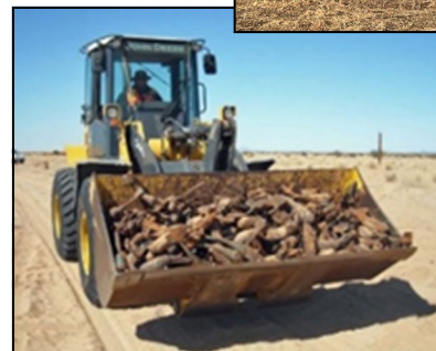
Large-Scale Debris Removal ←
