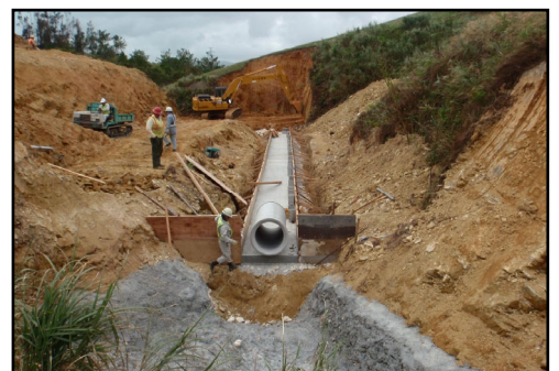
Range Drainage Improvements
