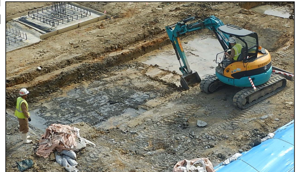
UXO Construction Support during soil operations, Okinawa, Japan
