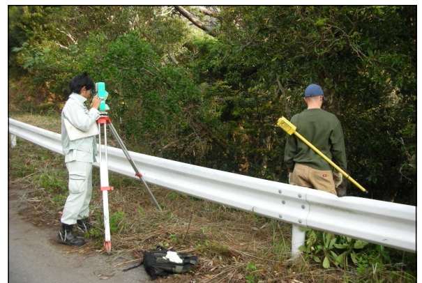
UXO Avoidance as Surveyors Plot Transects during Range Construction, Okinawa, Japan
