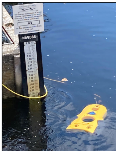
ROV being sent to inspect the inside of a SWFWMD culvert
