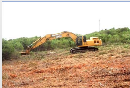
Robotic Vegetation Removal
