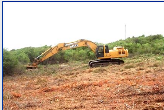
Robotic Vegetation Removal
